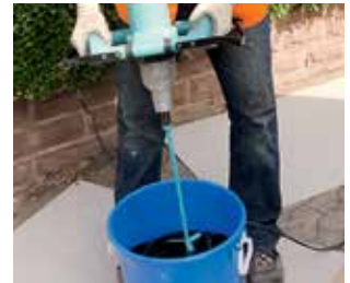
3. Mix Triflex Repro R and Triflex Asphalt Repro S well, then stir well with Triflex Catalyst for approx. 2 min.
