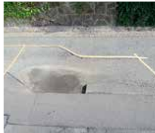
2. Tape off the area in need of repair.
