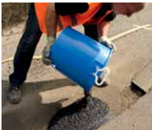
4. Transfer the mixed material to another receptacle and apply to the area in need of repair.
