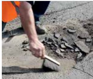
1. Remove dust and loose particles from the substrate.
