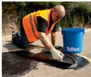
5. Spread and smooth the material with a trowel.
